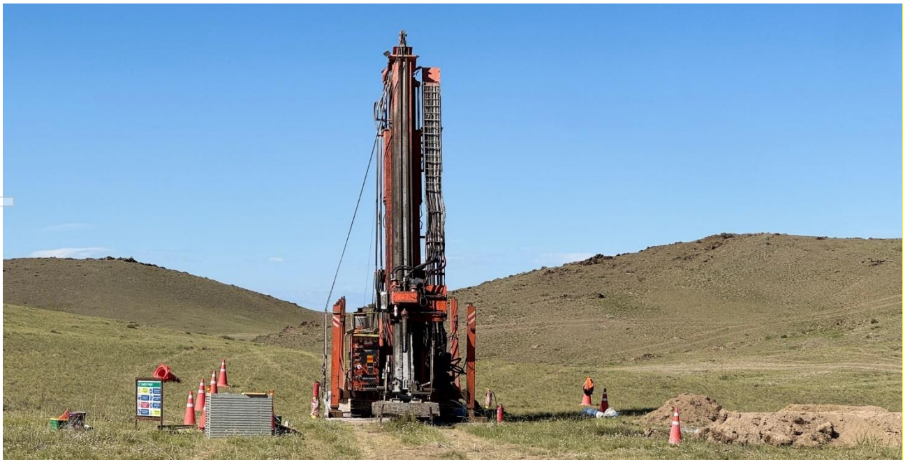
Photo 1. Phase 3 drilling of Oval Project – Aug 2025
